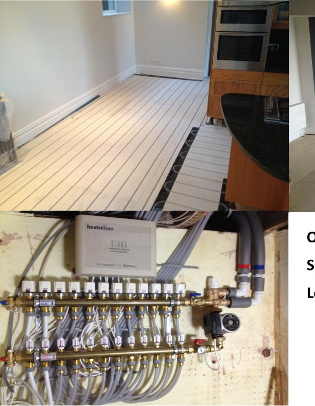
Overfloor underfloor heating system
